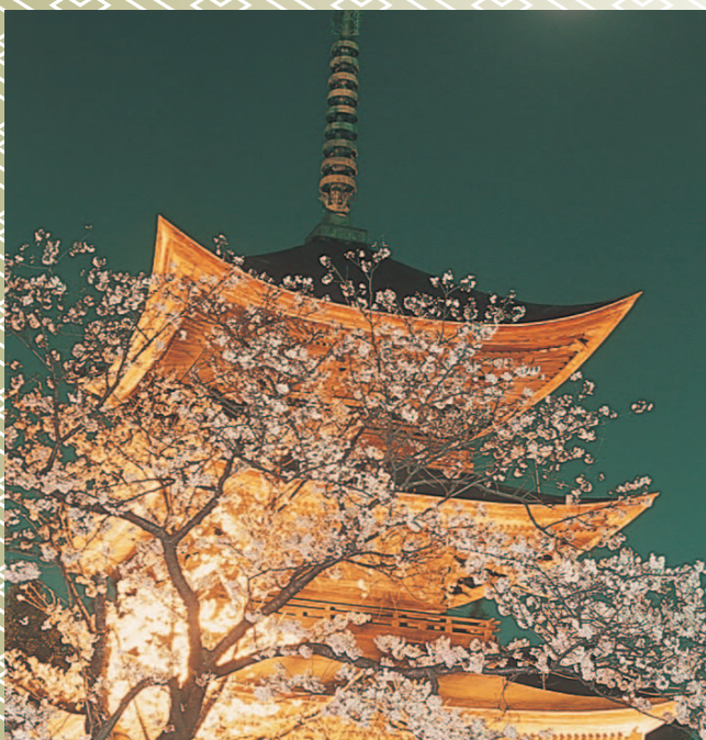
Three-story Pagoda at Sanmyoji Temple It is said that Sanmyoji Temple was constructed under the imperial rescript of Monmu Emperor. The first and second stories of the pagoda are in Japanese style, and the third story in Zen style. It is designated as a nationally important cultural property.
